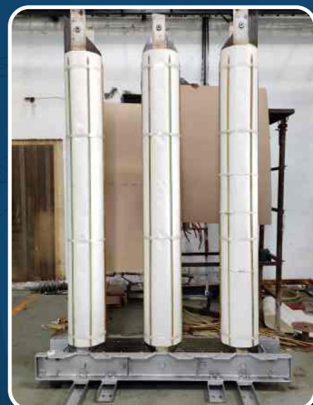
CORE AFTER CLEANING & REINSULATING
