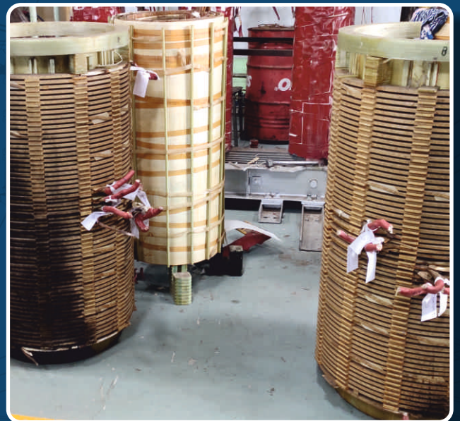
INDIVIDUAL COILS AFTER DISMANTLE
