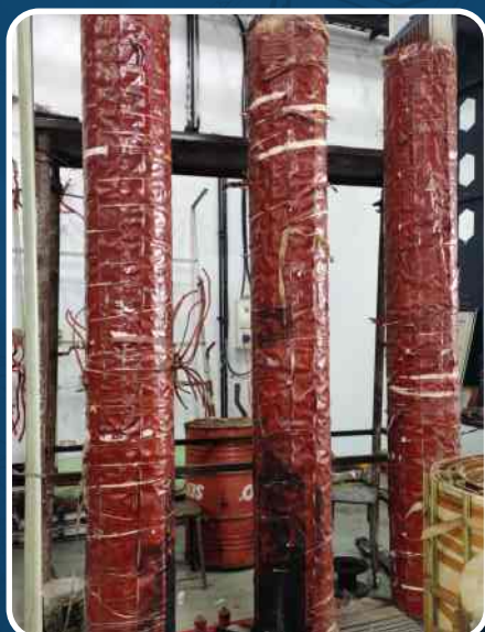
CORE BEFORE CLEANING & REINSULATING
